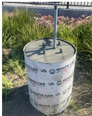
New caisson is poured.
