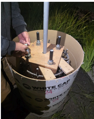
Raceway and bolts are aligned for new caisson.
