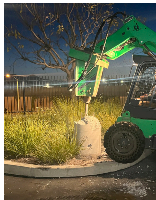
Caisson is demolished.
