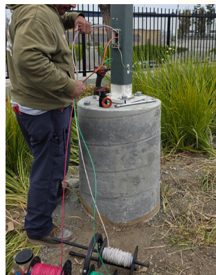
Light pole installed and wires pulled through.
