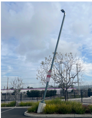
Light pole is clearly a hazard, needs removal.
