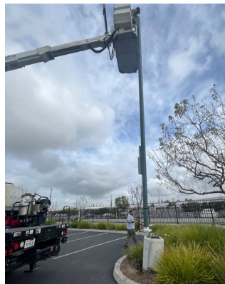
Light pole is removed from the caisson.
