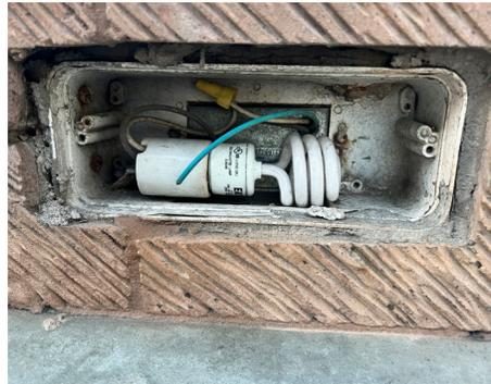
The way we solved this was to manufacture our own custom beauty plates. These plates cover the holes and simultaneously give the fixture something to mount onto. For added appeal, we powder coated the plates black.
