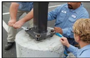
Level and Re-Secure Loose Nuts
